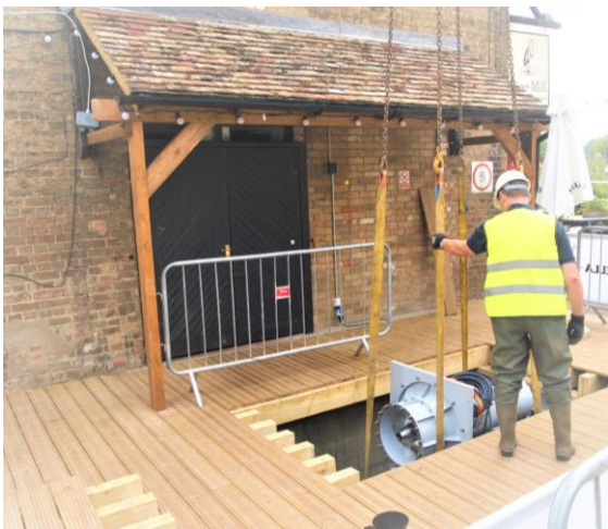
A VETT turbine during installation at Eaton Socon, Cambridgeshire in the UK.
