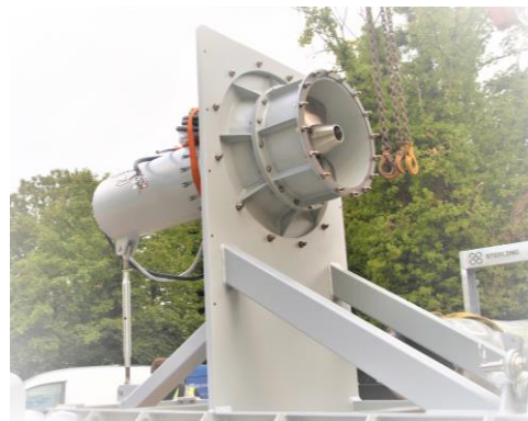
A VETT turbine-generator without draft tube during installation.
