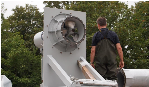
Figures 13-14: Installing the VETT turbine at Eaton Socon
