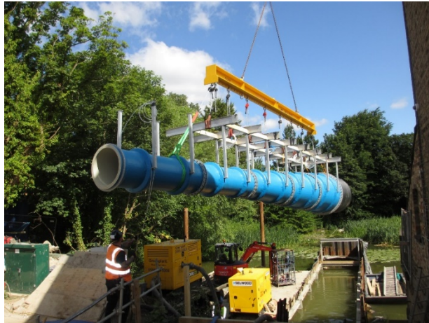
Figure 12: Installing the VETT pipe at Eaton Socon
