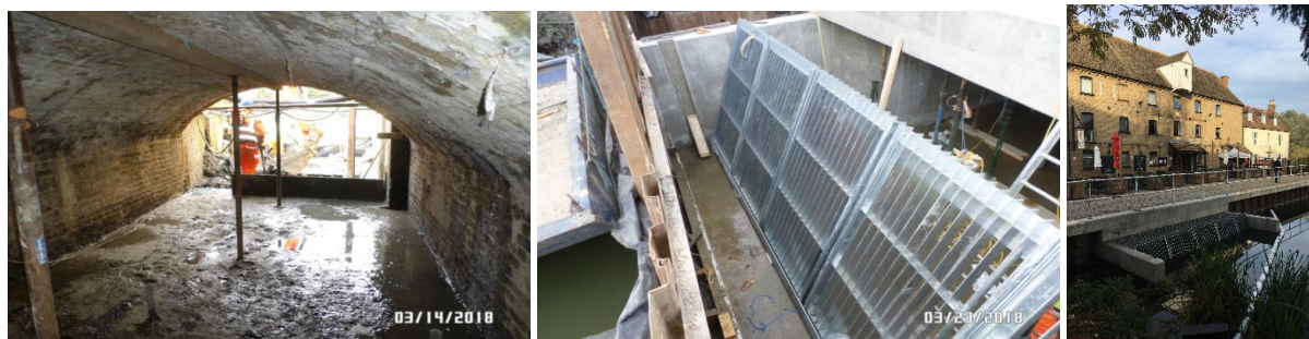
Figures 6-8: Photographs from the VETT installation at Eaton Socon showing the existing brick arch culvert and new intake and debris screen
